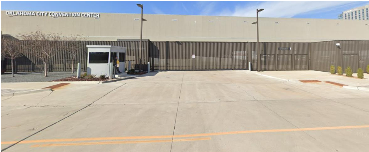
Loading Dock Entrance Gate, located on S Broadway Ave. near SW 5 th St.
